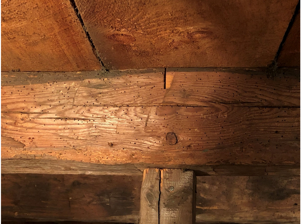
Fig. 5 Upper Loft Joist Notching
